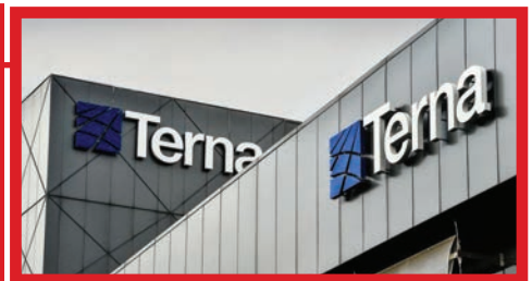
Data Center Terna (MI)
